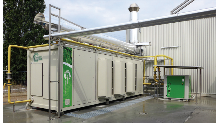
>> A Capstone C600 microturbine produces steam via post combustor for Aba Foods company in Italy
